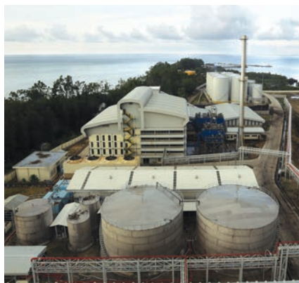
Palm Oil Refinery Indonesia
