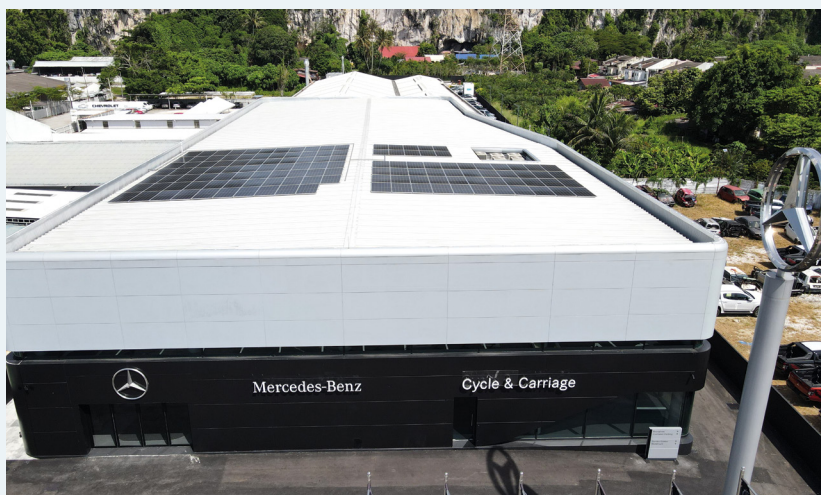
Rooftop solar at Cycle & Carriage Bintang Ipoh
