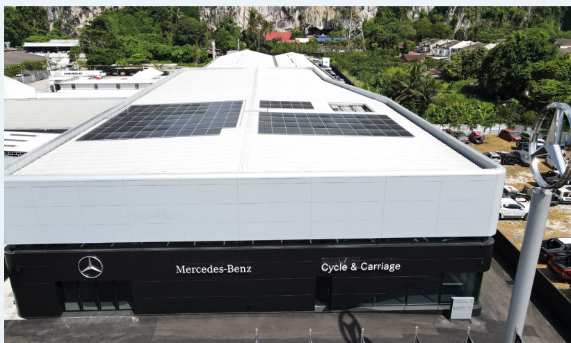
Rooftop solar at Cycle & Carriage Bintang Ipoh
