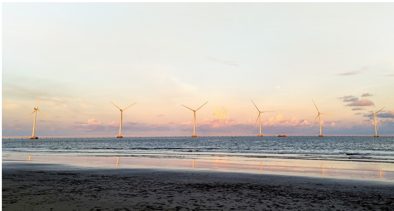
REE's Tra Vinh V1-3 Wind Power Plant
